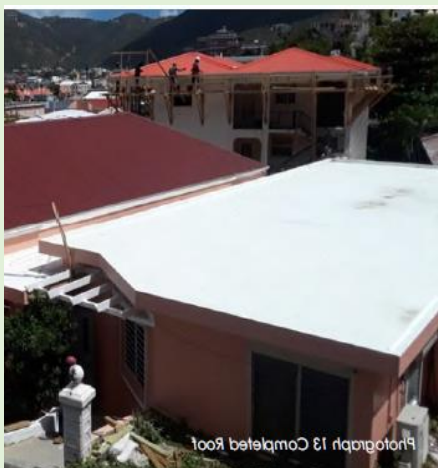
A: Roof painted white
